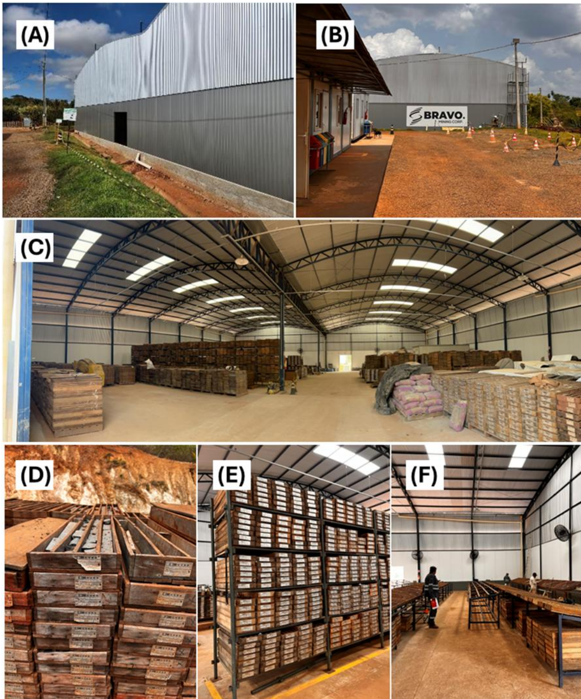
Figure 12-4: Core Shed installation during 1 st visit, and after complete construction on 2 nd visit
