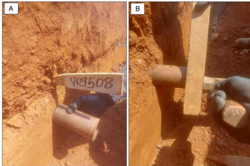
Figure 9-13: Cylinder insertion into weathered material
