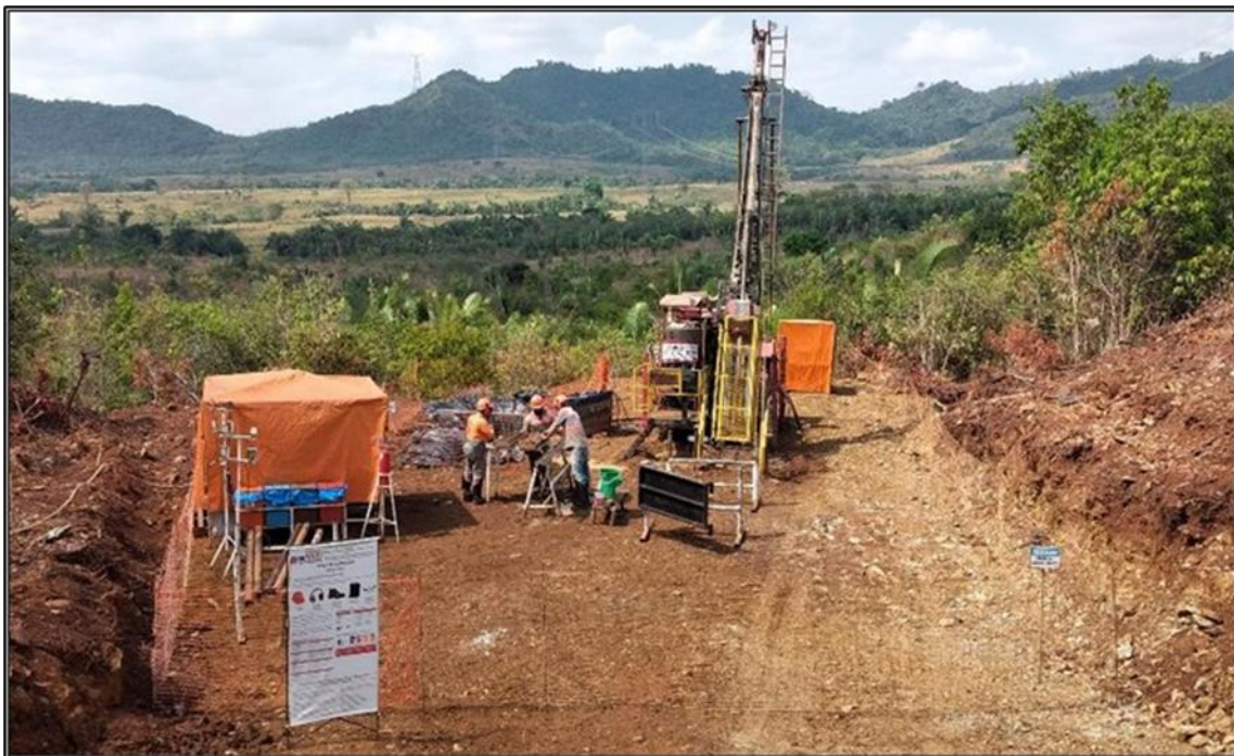
Figure 10-1: Drill rig in operation
