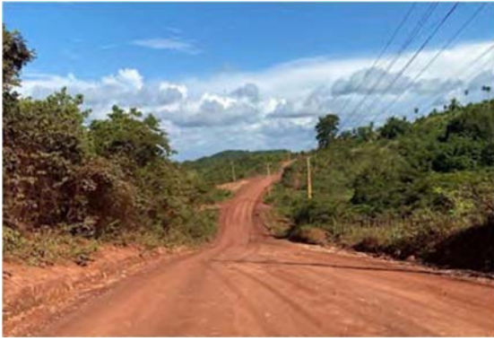
Unpaved Road to Site
