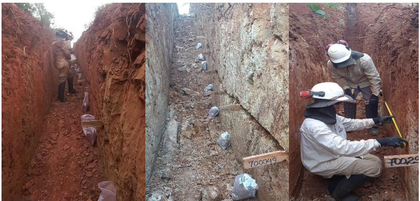
Figure 1: Trenching in the Southwest Sector.
