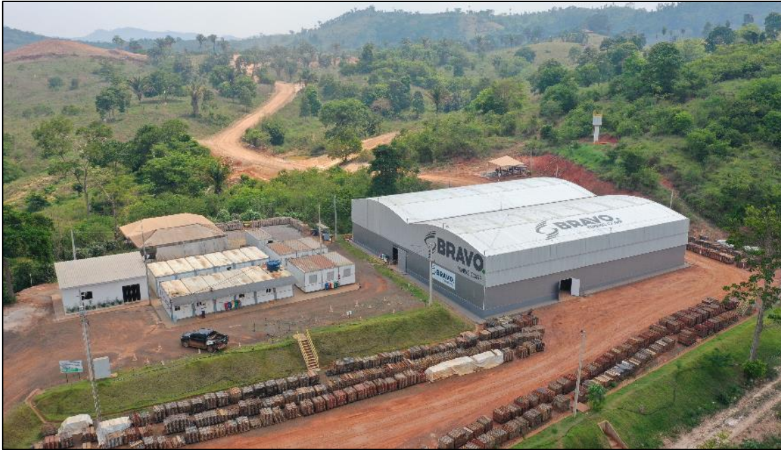
Figure 5-8: Bravo facilities at Luanga Project.
